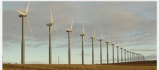
Stataline Wind Farm
