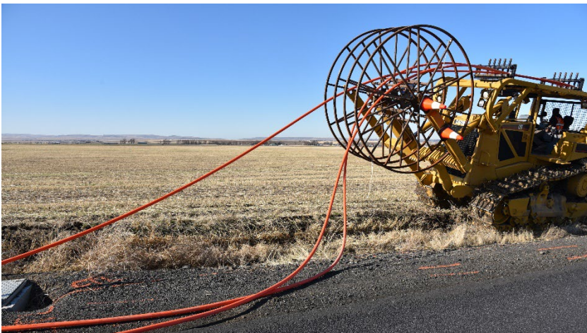
Coyote Business Park Fiber Optic Cable Installation ( CTUIR )
